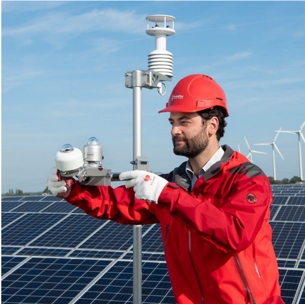
Figure 0.2 SR300-D1 includes a digital tilt angle measurement, a practical feature for remote verification of instrument mounting orientation. The above image depicts two SR300-D1 pyranometers, one tilted for Plane of Array (POA) measurement, and another mounted horizontally for Global Horizontal Irradiance (GHI) measurement.
